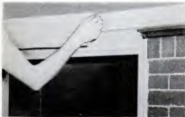
The plastic veneer is cut to size before application, as above. Application is not difficult and, if a little care is used, final appearance is like fine wood paneling. Below, mirror backs up small shelf
